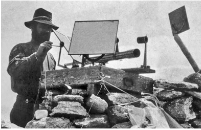
b / A surveyor on a mountaintop uses a heliotrope.
